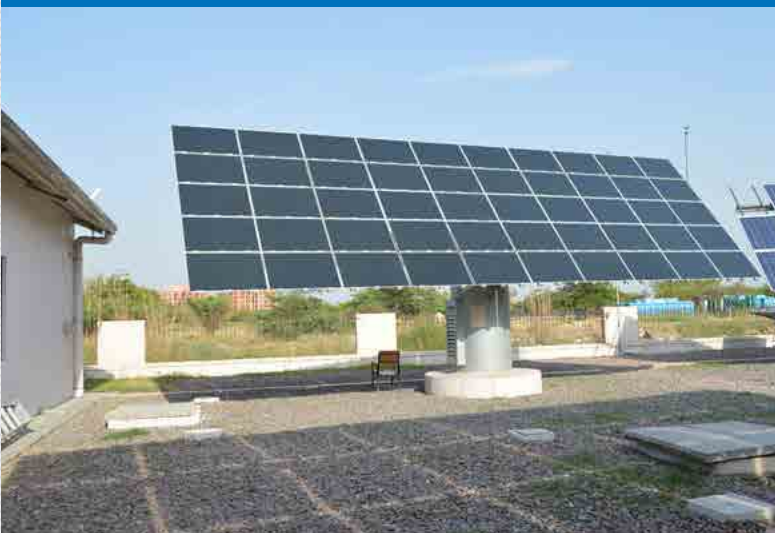
Solar Energy Research Enclave, IIT Kanpur
